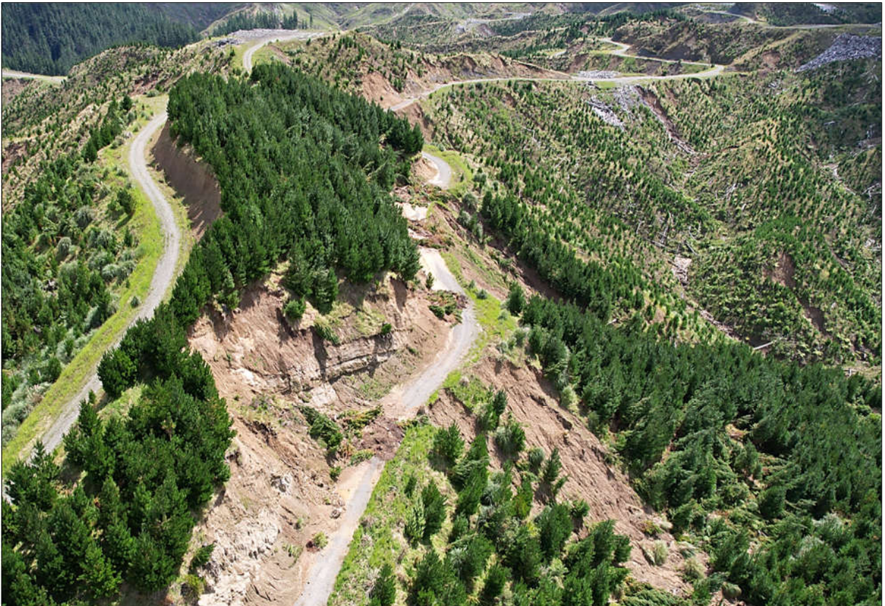
Photo 3: Roads in Hokoroa Group forests, Gisborne damaged by flooding, and soil loss below the road (photo March 2023).
