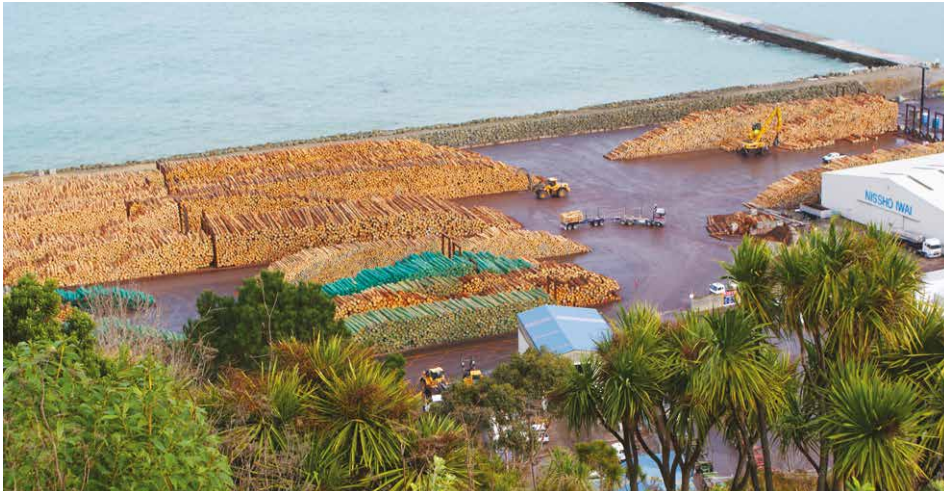
Eastland Port in Gisborne is the third busiest wood export port in Aotearoa New Zealand, handling nearly three million tonnes of logs a year, and scheduled to double this over the next few years
