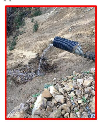
Culvert outlets must discharge onto stable ground. Discharge over fill must be flumed (plastic or PVC sock) where PVC socks are used these must be installed eyelet down and attached to ground (as per manufacturer's instructions).
